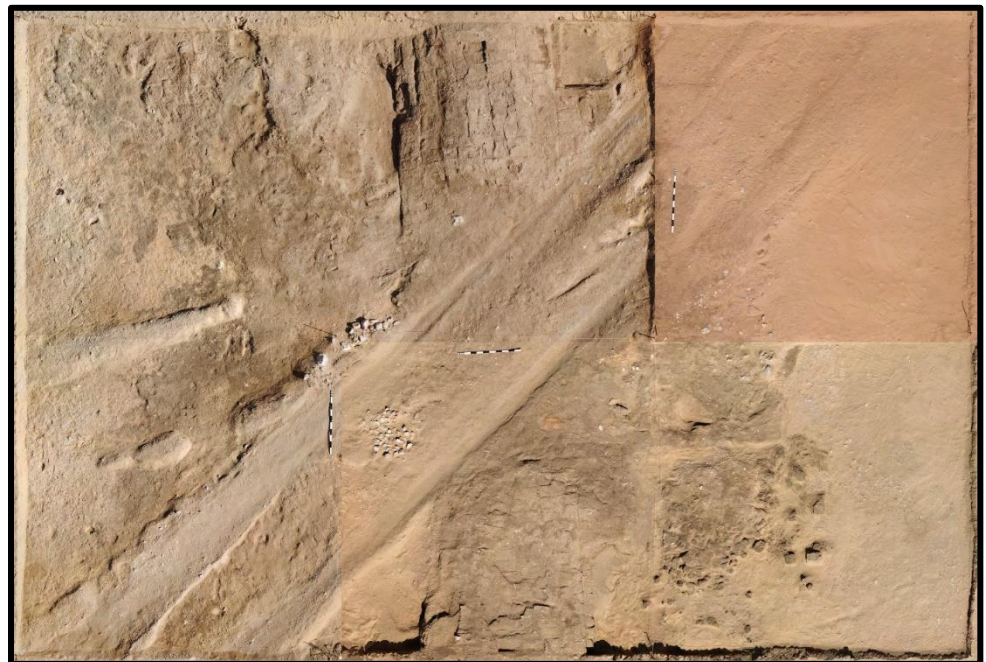
Figure 21: Collage of aerial photographs taken in 2021 and 2022 showing the tyre tracks damaging the East Gateway. Orthomosaics by Fabien Balestra.
